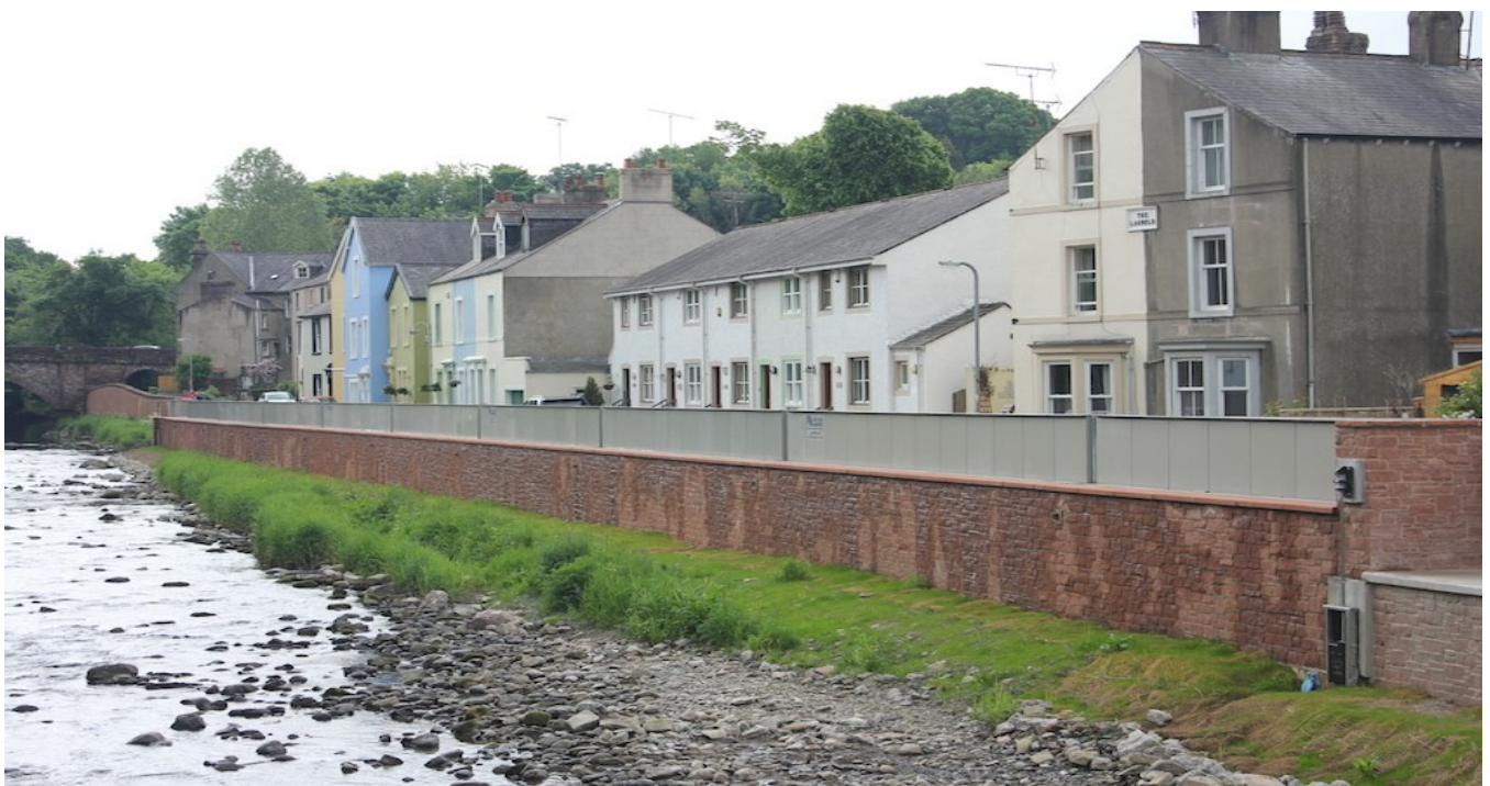
123 meter SCFB 1000 protection of the town Cockermouth in the UK
